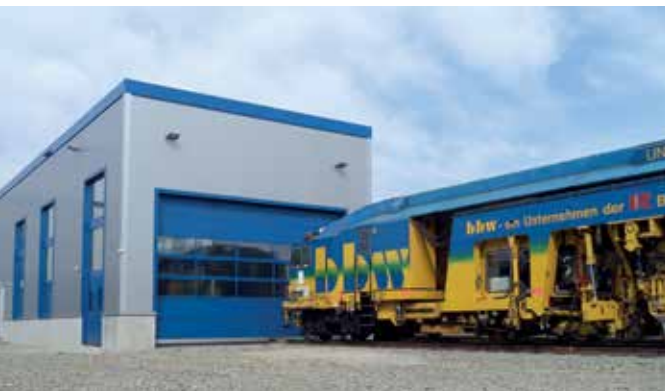
Expansion on the Bahnbau Wels company site: the new building is available for maintenance work and winter repairs.
