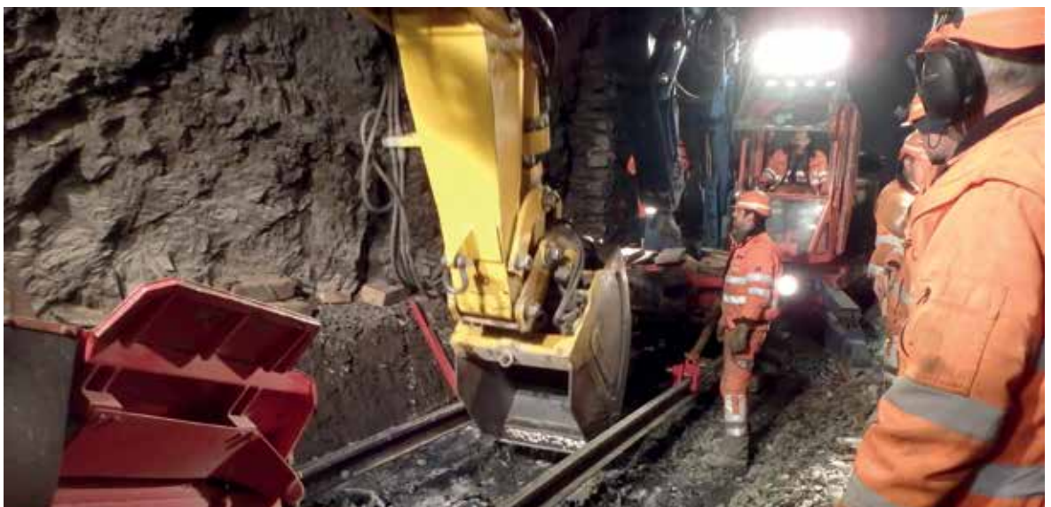
Lowering a track using the special TYREX metre gauge machine.
