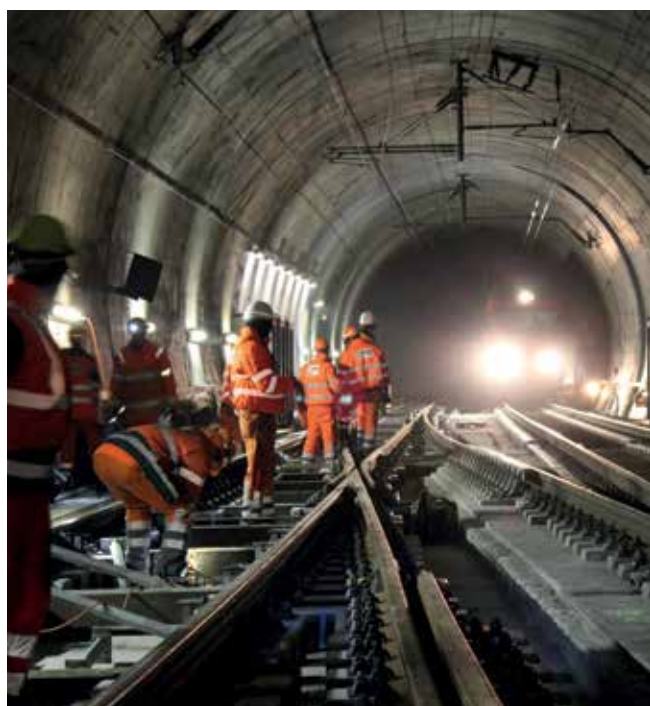
Workers during the alignment of a switch point.
