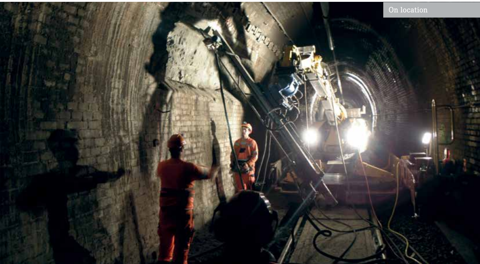
Producing a 60° bar anchor, middle section (collar niche 2, Simplon tunnel IIb).
