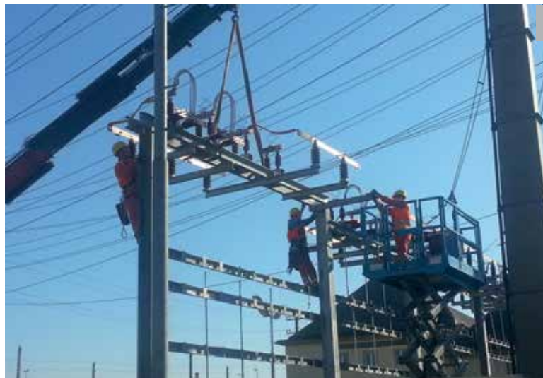
Installation of a switch frame at Amstetten railway station, Austria.
