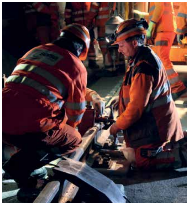
Preparation for rail welding work.
