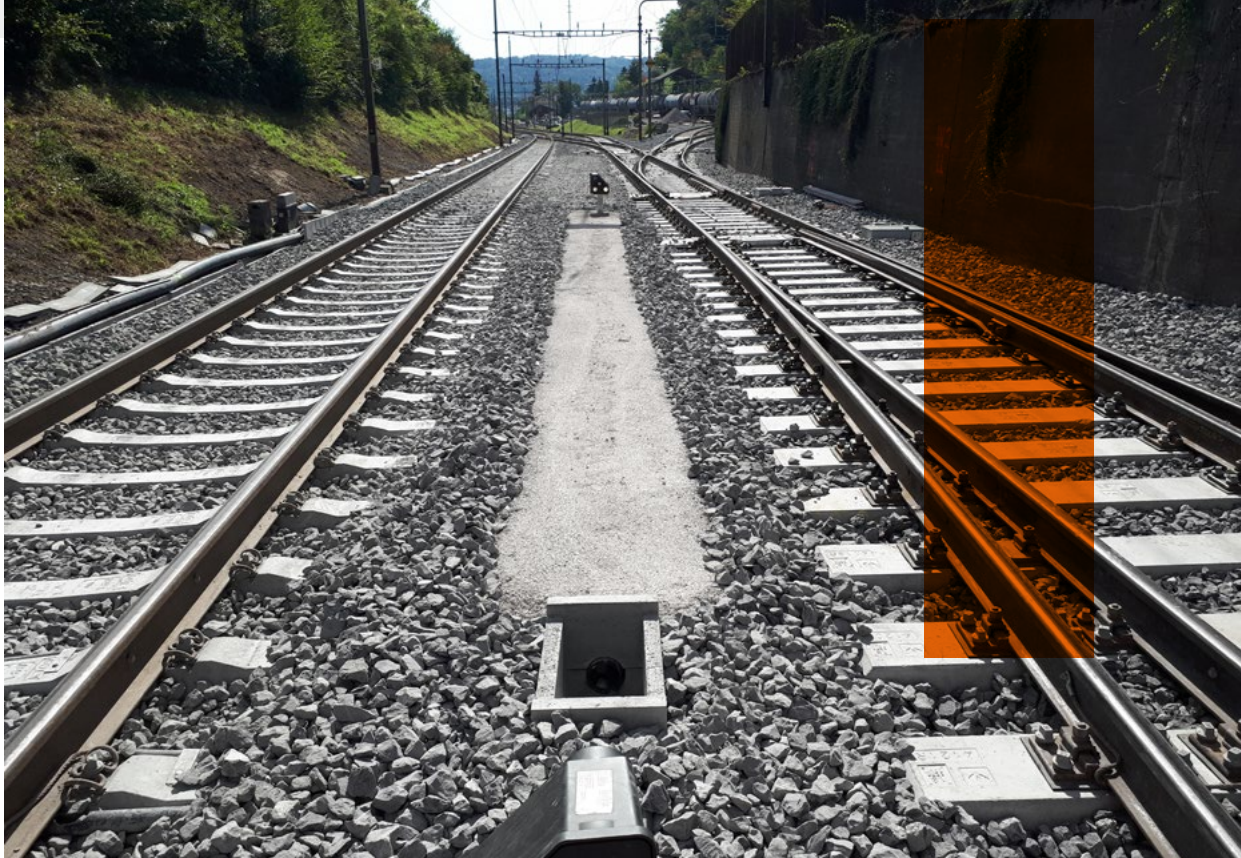
Completed track construction
