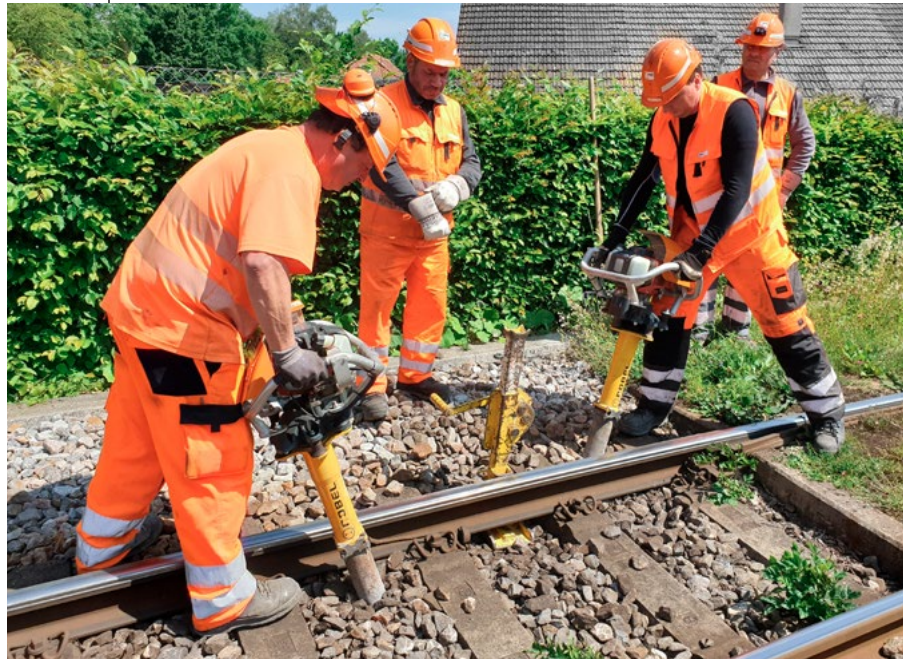
Elimination of individual faults in Auzelg
