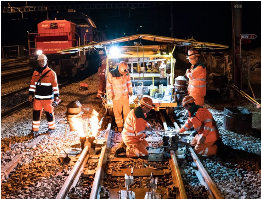
■ Aluminothermic welding at switches
