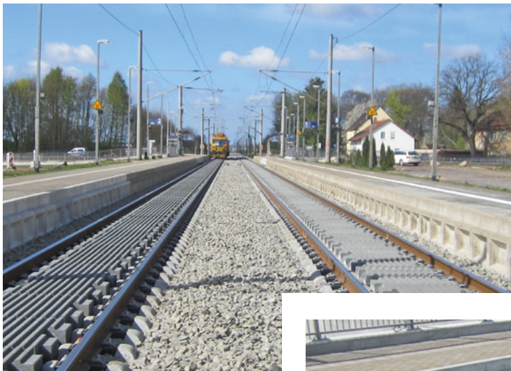
After a warm winter the trains now run on slab track.
