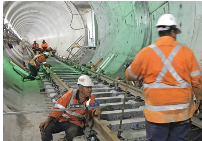
...of the installation of slab track in Australia's longest railway tunnel.
