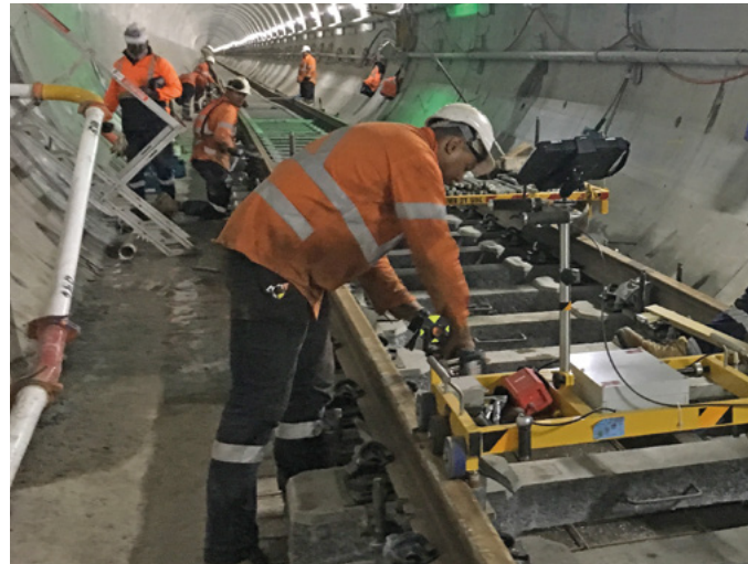
Slab track down under – down under Sydney: impressions...
