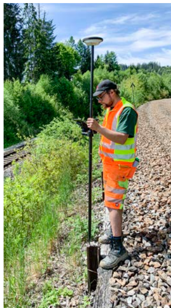
Employee Christian Henisch sets survey stations using a GNSS positioning antenna
