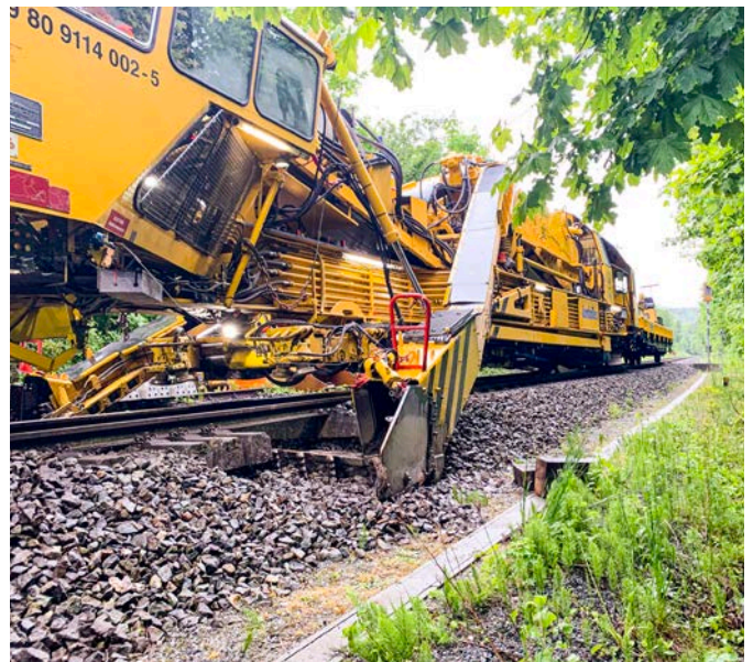
Ballast screening machine RM 80-92 UHR on the Deggendorf-Ulrichsberg line (JumboTec)
