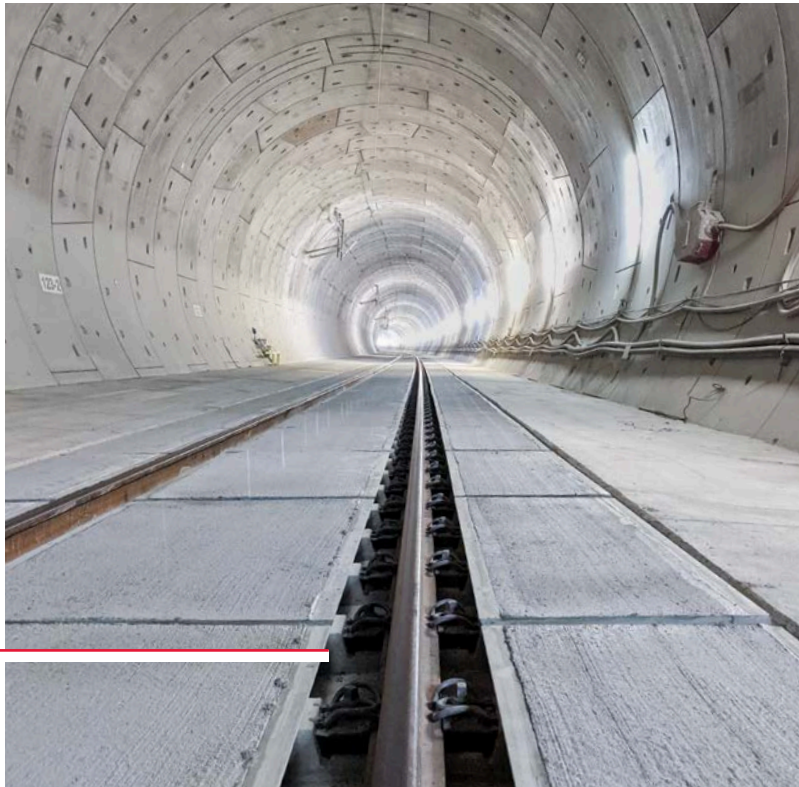
The in-house development of level crossing segments for slab track systems allows access for road vehicles.
