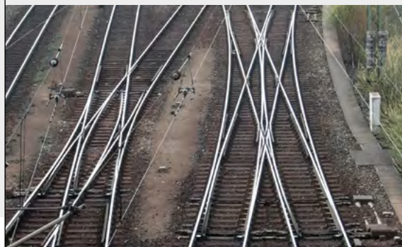
In direct comparison: double slip switches with inside (pictured left) and outside switches (pictured right)
